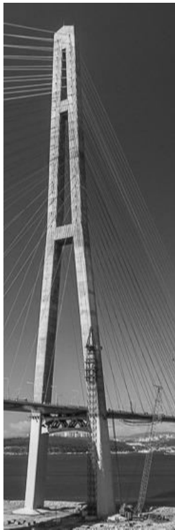
Fig.3. Rusky Bridge Pylon. ( https://structurae.net/en/structures/rusky-bridge ) [5]
