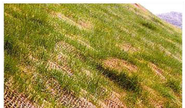
Geotextile coating with plantation
