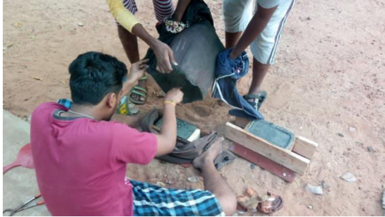
Fig 4 Casting of plasto pavers.
