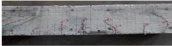
Figure 12. Crack Pattern for Optimum Mix Beam
