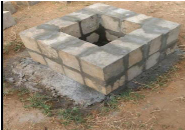
Fig 5.5 Basement using concrete cubes
