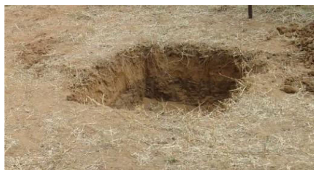
Fig 5.3: Site Excavation for Proceeding our Installation Work
