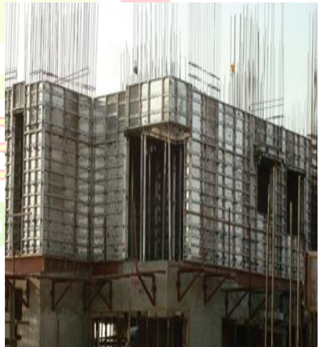
Figure 4 – centering and shuttering
