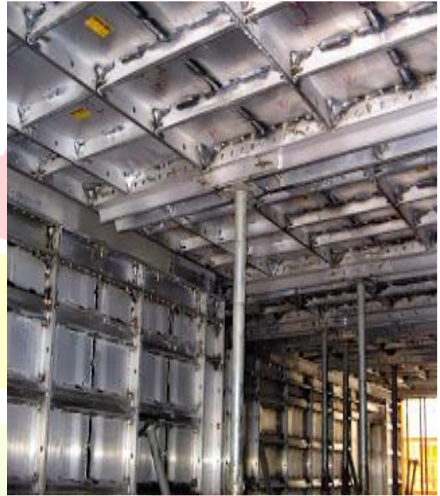
Figure 4 – centering and shuttering
