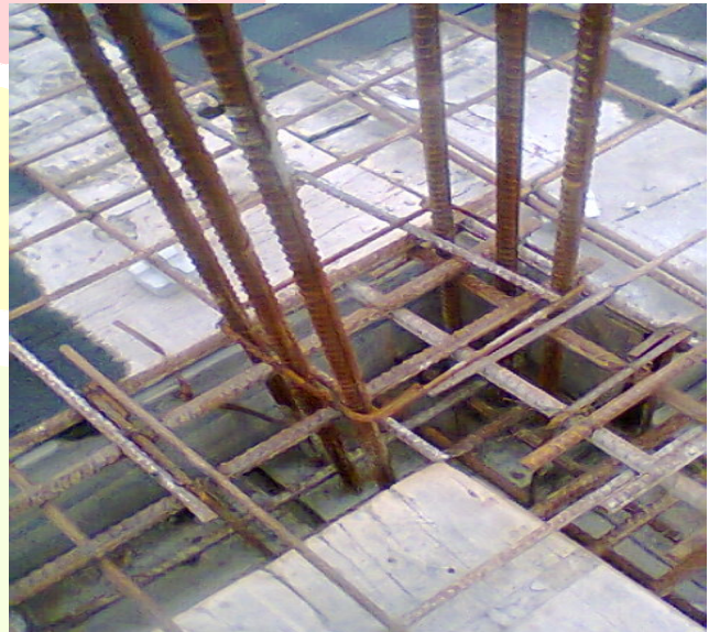
Fig.1. Beam – column joint at corner
