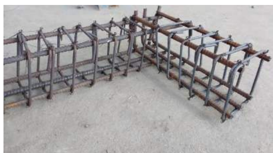
Beam B reinforcement detail
