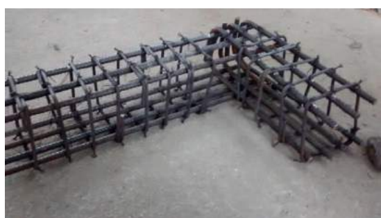
Beam A reinforcement detail
