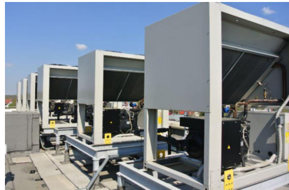
Picture :1: Chillers installed on a roof
