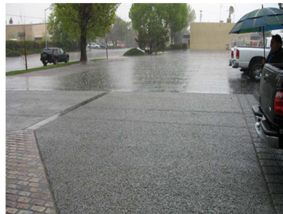
Fig 1.4 Parking area of pervious concrete
