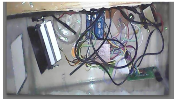
Fig(6) Complete system work
